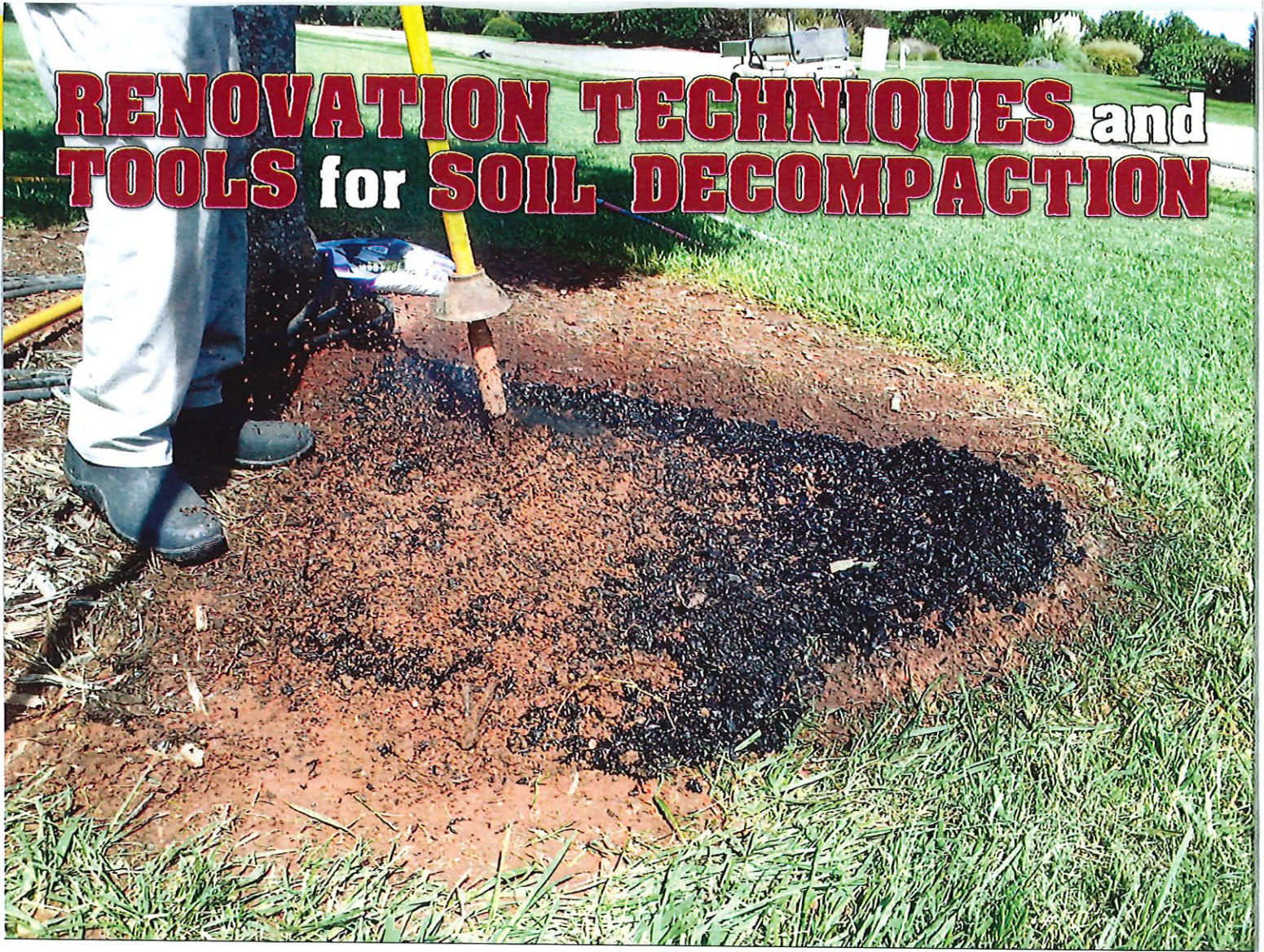
Biochar being incorporated into existing soil with a pneumatic air tool. Photos courtesy of the author, unless otherwise specified.
